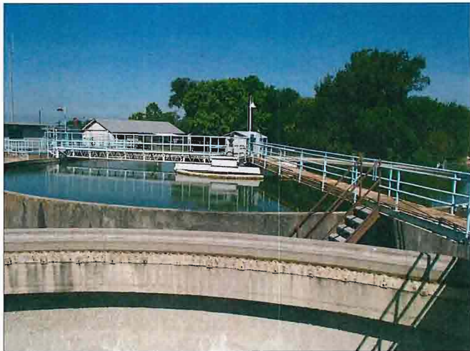
CLARIFIER No. 1 FROM CLARIFIER No. 2
