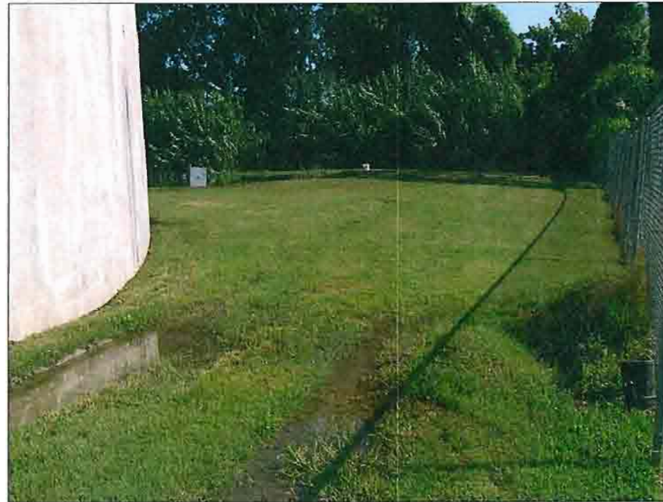
6" RECYCLE LINE (EAST SIDE OF CLARIFIER No. 2)
