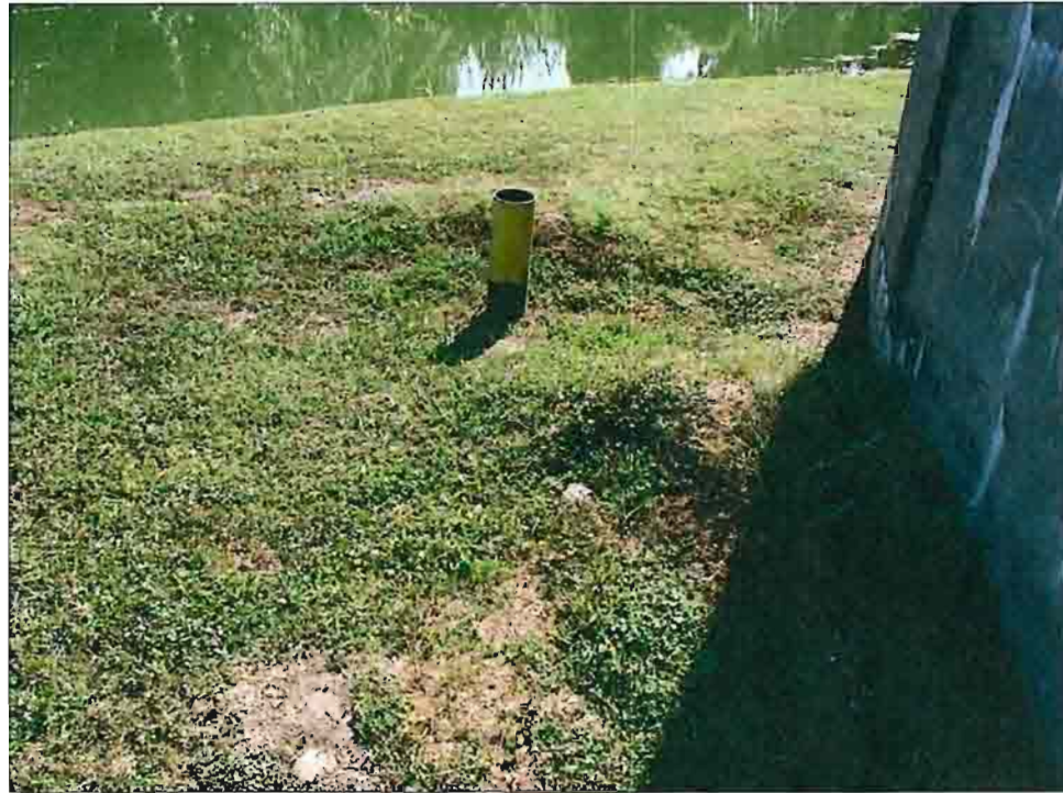
CLARIFIER No. 2 6" SLUDGE VALVE RISER BOX
